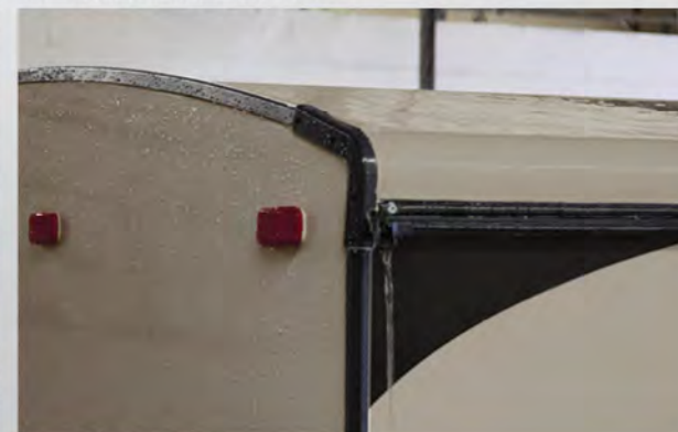
TPO Roll Over Roof
